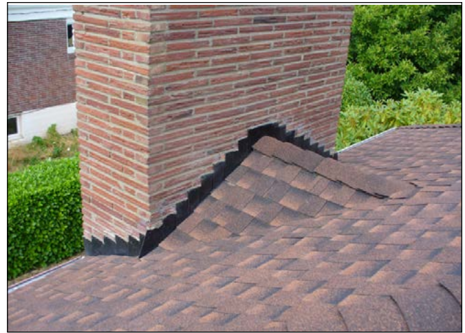
Cricket or saddle at chimney.
