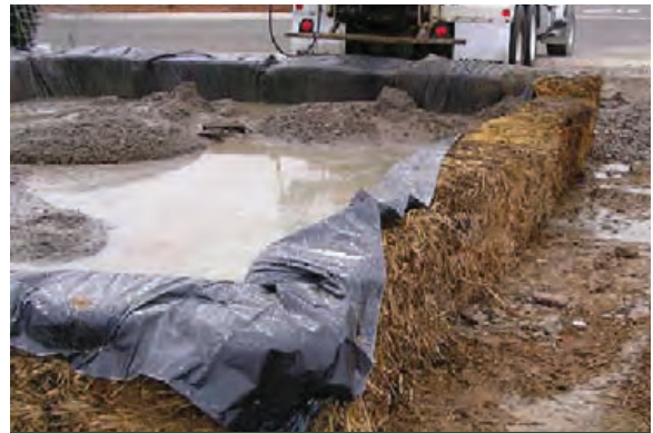
Concrete Washout
