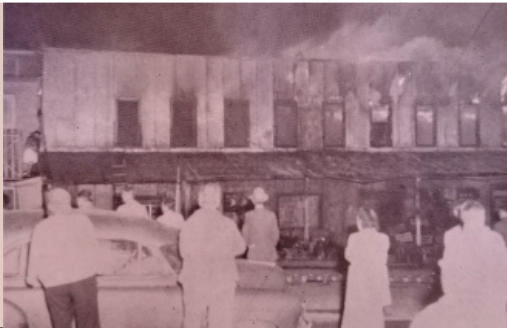
Stork Bros. Plant fire 1953 CITY OF NEW ULM PHOTO
