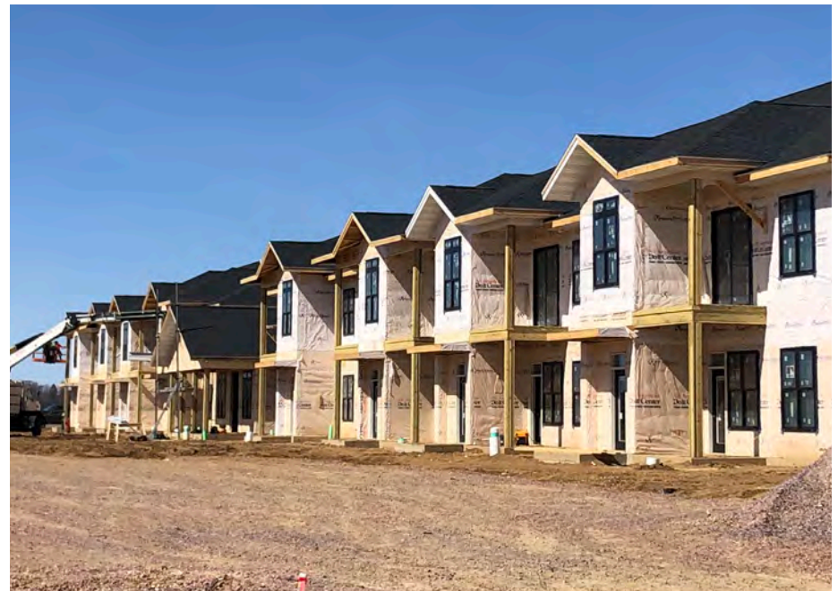
Example of new construction being built
