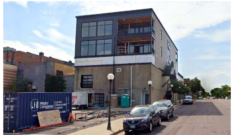
New multi-use building with upper level housing being built in Downtown
