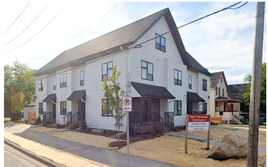
Example of new townhomes built in a residential neighborhood
