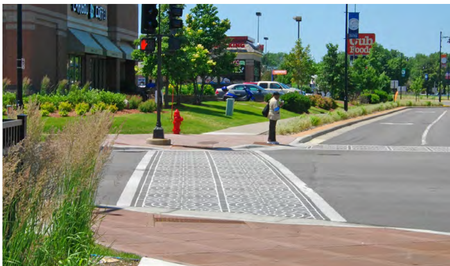
Example of marked crosswalk to improve visibility of pedestrians in a commercial area
