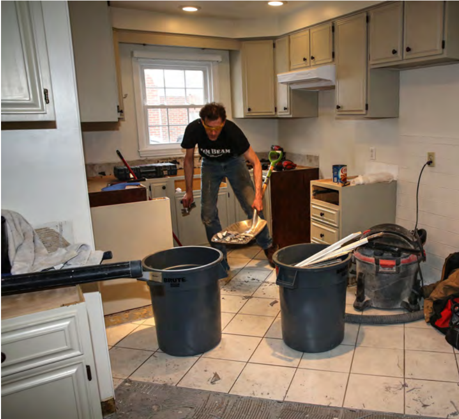
Example of indoor rehabilitation
