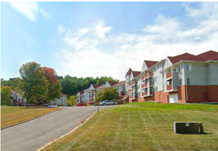
Garden Terrace Apartments
